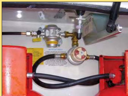
Option 2 Fit an 01-1755 automatic changeover head.
