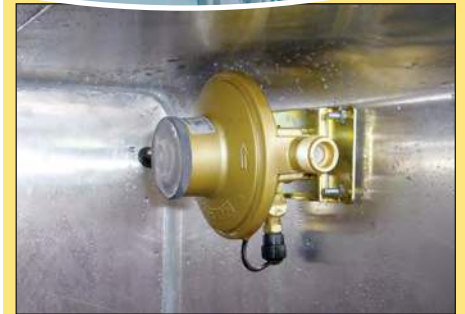
Typical configuration with Regulator in top right and inlet facing you.
