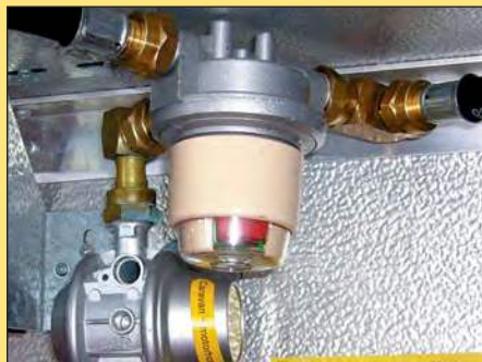
Option 2 Loosen and rotate the pre fitted elbow 30 degrees - Fit an 01-1755 automatic changeover head. Notice we have used a 01-1677 on the right outlet due to the restriction of the back wall
