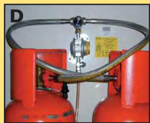
Picture shows a Truma regulator upgraded to a manual changeover with a 01-1630 and using two propane 0.75 meter Stainless hoses. Note how the hoses cross preventing unnecessary kinking and twisting.
